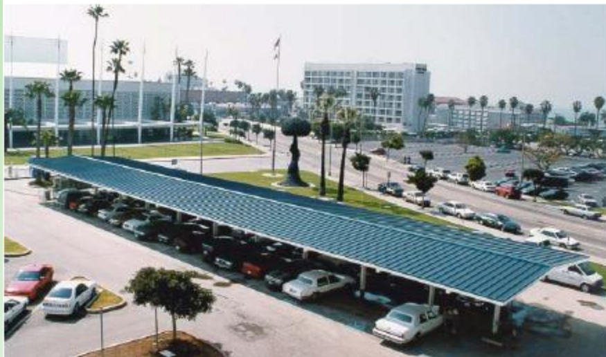
30 kW EV Charging Shade Structure
